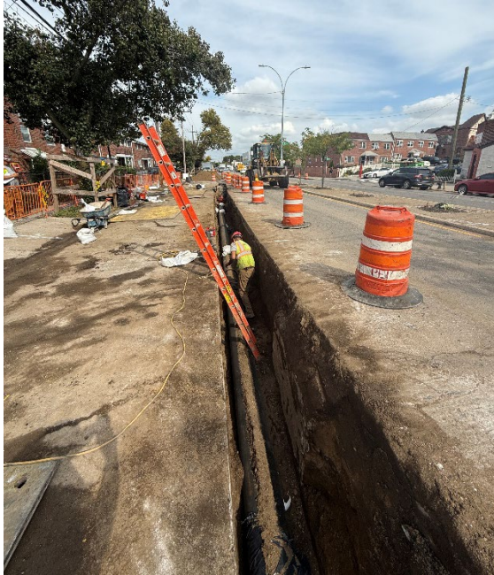
Springfield Boulevard water main installation
