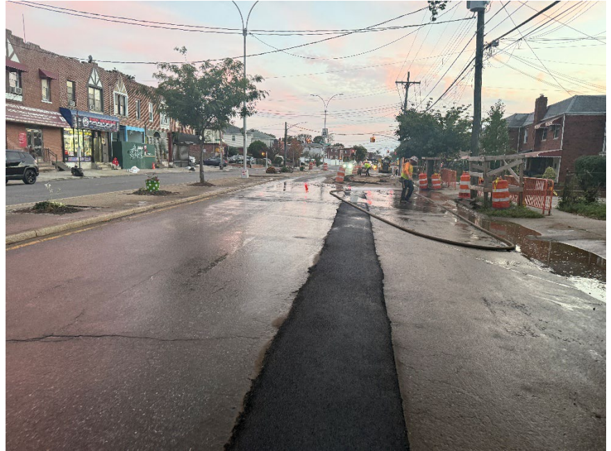
Springfield Boulevard water main installation
